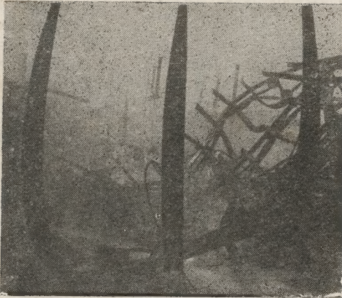
Like the teeth of a gigantic pitchfork, three steel girders rest on the floor of the Esso Club lobby the morning after the fire.
